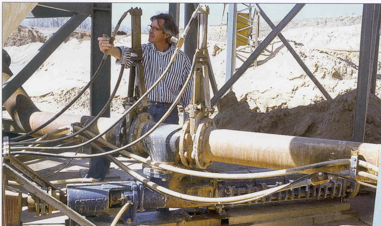
The author inspects a progressive cavity pump used in Clearwater Industries' water clarification system in service at John Sand & Gravel Co., in New Berlin, Wisconsin.
